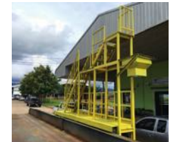
Install stairs and handrails
