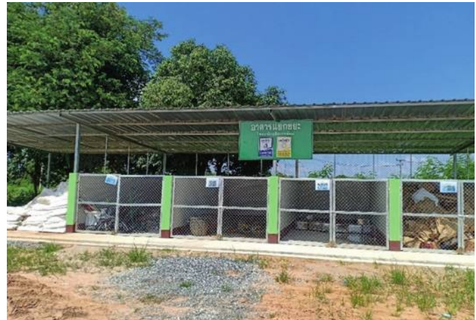
Waste sorting building
