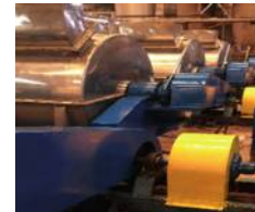
Install the machine pivot point guard
